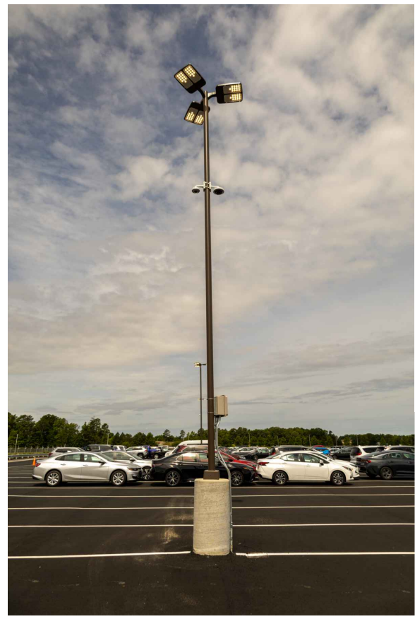
AREA LIGHTING: TRIPLE LED LUMINAIRE TO MATCH AIRPORT STANDARD. COLOR: WHITE
